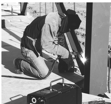
Figure 1 FCAW-S in Building Construction
